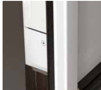
Astragal bolt penetrates threshold allowing boot to seal, creating a better barrier against the elements
